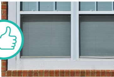
DOUBLE-PANED WINDOW, INSTALLED WITH PROPER FLASHING
