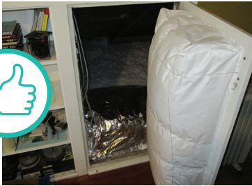
WEATHERSTRIPPED AND INSULATED HATCH
