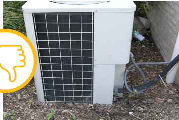
OUTDOOR UNIT SET DIRECTLY ON THE GROUND
