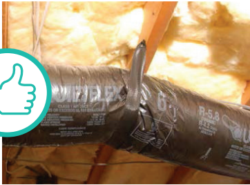
DUCT PROPERLY SUPPORTED
