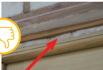
INCOMPLETE SEAL AROUND NEWLY INSTALLED WINDOW
