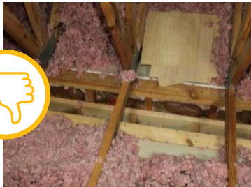
OPEN/UNSEALED CHASE OR CAVITY
