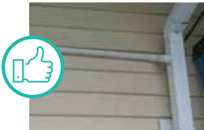
CONDENSATE DRAIN IS CONNECTED TO DOWNSPOUT Courtesy of NW Ductless Heat Pump Project
