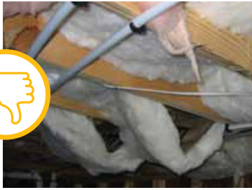
INSULATION DOES NOT FILL CAVITY AND NOT PROPERLY SUPPORTED
