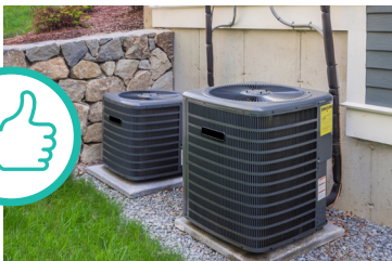
OUTDOOR UNIT INSTALLED IN CLEAR AREA THAT ALLOWS OPTIMAL AIRFLOW THROUGH FAN
