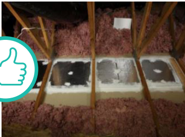
SEALED CHASE OR CAVITY
