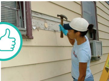
INSULATION ACCESS HOLES PLUGGED AND SEALED WITH SOLID PLUGS Courtesy of U.S. Department of Energy
