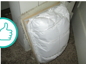
CRAWL HATCH INSULATED AND WEATHERSTRIPPED
