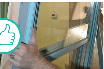
PROPER FIT WINDOW, LEVEL, AND SEALED
