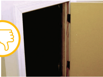
UNINSULATED, NOT WEATHERSTRIPPED
