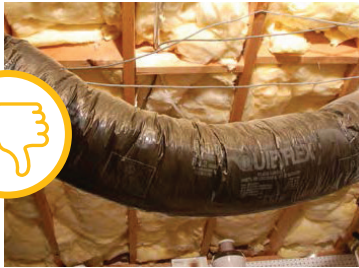
DUCT IS NOT PROPERLY SUPPORTED
