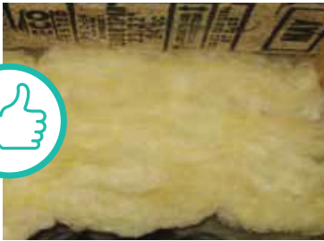
INSULATION IN FULL CONTACT WITH FLOOR
