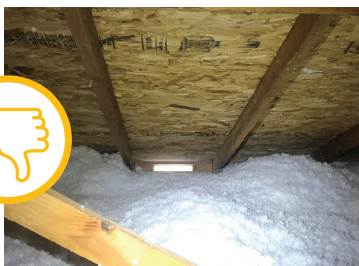
ROOF-TO-WALL HEEL UNINSULATED
