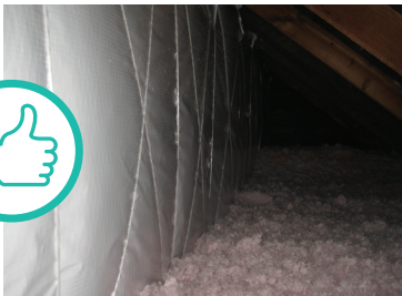
OPEN KNEE WALL INSULATED AND COVERED
