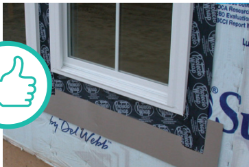
PROPER FLASHING WINDOW TO WEATHER BARRIER
