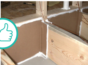
FLOOR JOISTS UNDER KNEEWALL
