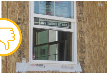
IMPROPERLY FLASHED WINDOW
