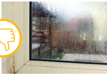
UNINSULATED WINDOW WITH CONDENSATION
