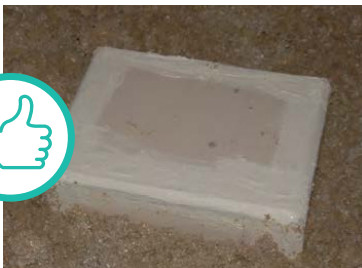
NON-IC FIXTURE WITH DRYWALL SHIELD (HAT)
