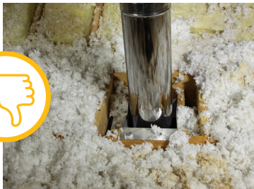
UNSEALED PENETRATION (HEAT-PRODUCING)
