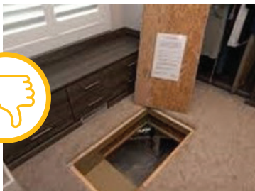
CRAWL HATCH NOT INSULATED
