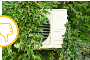
OUTDOOR UNIT INSTALLED IN A CONSTRAINED AREA THAT LIMITS OPTIMAL AIRFLOW THROUGH FAN
