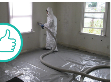
INSULATING BRICK OR STUCCO WALL FROM INTERIOR Courtesy of South Seattle Community College
