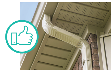
INSPECT ALL DOWNSPOUTS FOR PROPER CONNECTION
