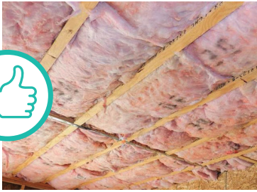
INSULATION FILLS CAVITY, PROPERLY SUPPORTED
