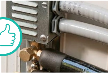
ALL LINE SET/REFRIGERANT LINES PROPERLY INSULATED Courtesy of PTCS
