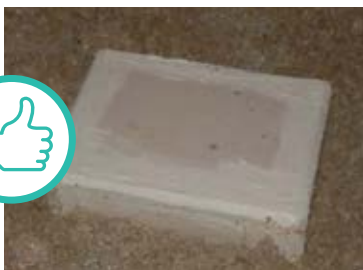
NON-IC FIXTURE WITH DRYWALL SHIELD (HAT)
