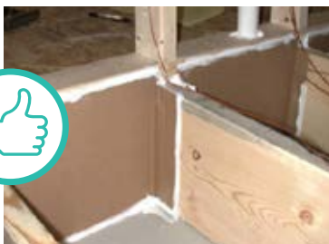
FLOOR JOISTS UNDER KNEEWALL
