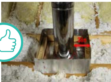
SEALED PENETRATION (HEAT-PRODUCING)
