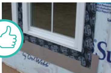
PROPER FLASHING WINDOW TO WEATHER BARRIER
