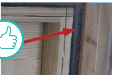
BACKER ROD AND CAULK COMPLETE SEAL AROUND WINDOW FRAME
