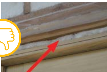
INCOMPLETE SEAL AROUND NEWLY INSTALLED WINDOW
