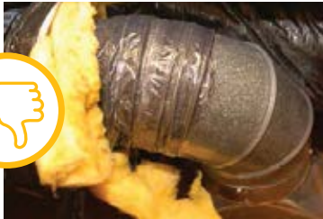
FLEX DUCT IS NOT MECHANICALLY FASTENED TO METAL DUCT
