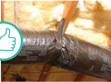
DUCT PROPERLY SUPPORTED
