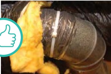
FLEX DUCT IS PROPERLY FASTENED TO METAL DUCT WITH MECHANICALLY TIGHTENED STRAP
