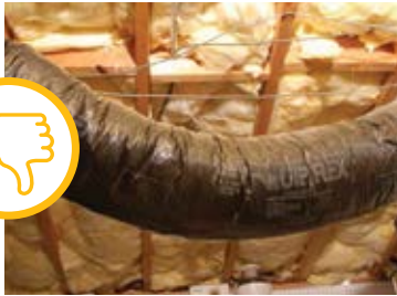
DUCT IS NOT PROPERLY SUPPORTED
