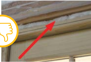
LOOSE-FILL INSULATION ALLOWS MOISTURE AND AIR INFILTRATION Courtesy of U.S. Department of Energy
