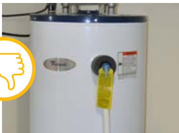
DOES NOT MEET MINIMUM EFFICIENCY Courtesy of Santa Fe Community College
