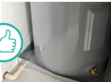
DRAIN PANS CAN HELP PREVENT MESSSES AND WATER DAMAGE
