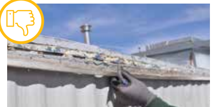
Gutter not properly attached, potential leaks at roof edge. Courtesy of Santa Fe Community College
