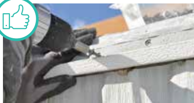
Edge of roof secured and gutter re-attached. Courtesy of Santa Fe Community College
