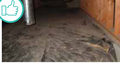
Clean crawl, good ground cover. Courtesy of Oregon Housing and Community Services and Oregon Energy Coordinators Association
