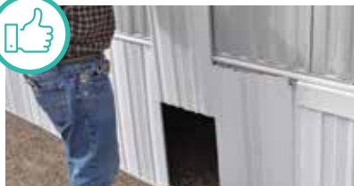
Properly fixing skirting. Courtesy of Santa Fe Community College
