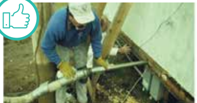
Insulating belly from edge fill method. Courtesy of U.S. Department of Energy
