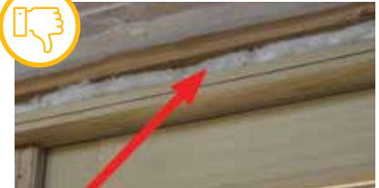
Loose-fill insulation allows moisture and air infiltration. Courtesy of U.S. Department of Energy
