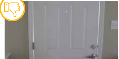
Bad air leaks around door. Light is visible in the cracks. Courtesy of U.S. Department of Energy
