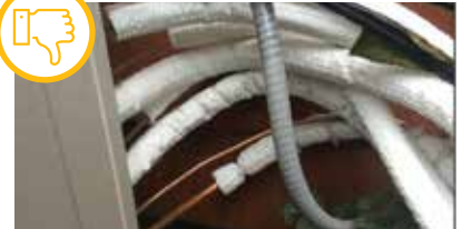
Line set/refrigerant lines not completely insulated.
