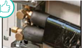
All line set/refrigerant lines properly insulated.
